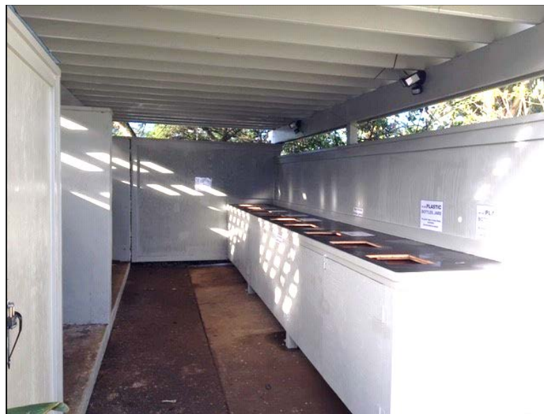
Expanded recycling center adjacent to building 4
