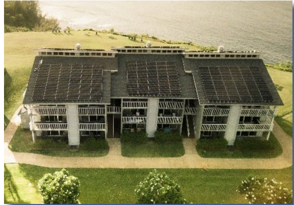
Roof-mounted photovoltaic panels provided 79% of the total electric demand on the property in 2022
