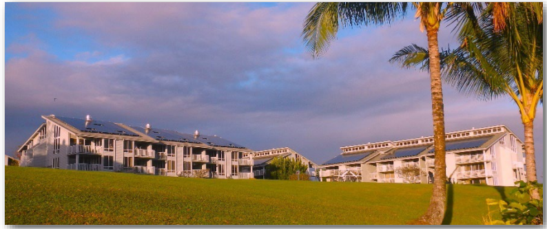
Residential buildings perched on the ocean bluff provide guests and residents with spectacular ocean vistas.
