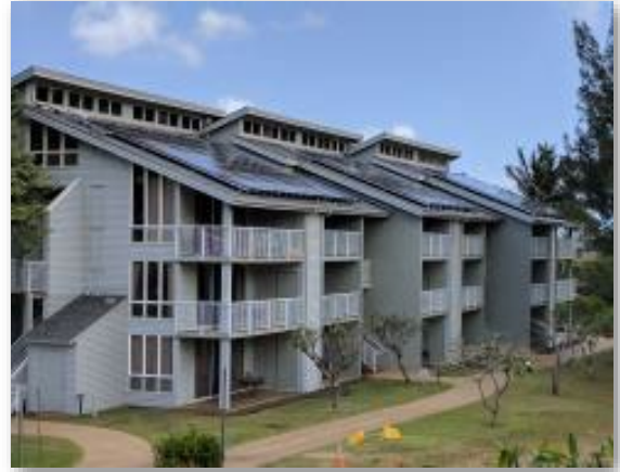
Roof-mounted solar panels generated 74% of the total electricity demand for the property in 2023
