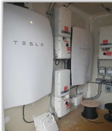
Tesla Powerwall batteries provide for storage of excess renewable energy generated during daylight hours and used at night
